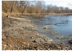
Woody debris and rock installed for aquatic habitat and bank protection.
