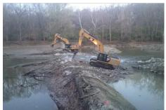
Excavators removing 300' wide dam.
