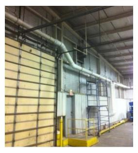
New roof drain lines from internal roof gutters increased capacity and prevents flooding in the building.
