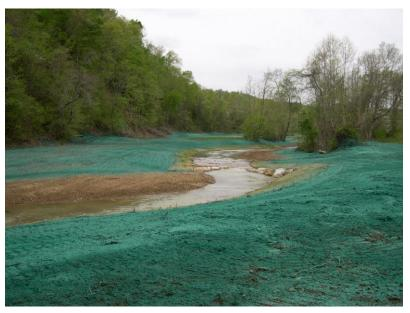
and perennial native grass and wildflower seed was applied in the spring of 2005. The advantage of hydroseeding was that the seed slurry also included tacifier and cellulose pulp. The tacifier was formulated from a natural gum to help hold soil particles together as well as help the cellulose pulp adhere to the steep slopes. The wet cellulose acted as a spongy media to facilitate seed
